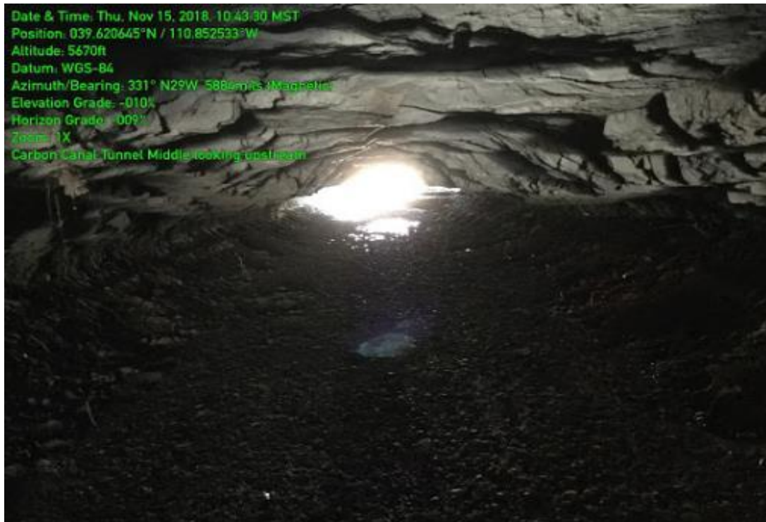
Figure 5. Interior view of tunnel looking upstream. November 15, 2018
