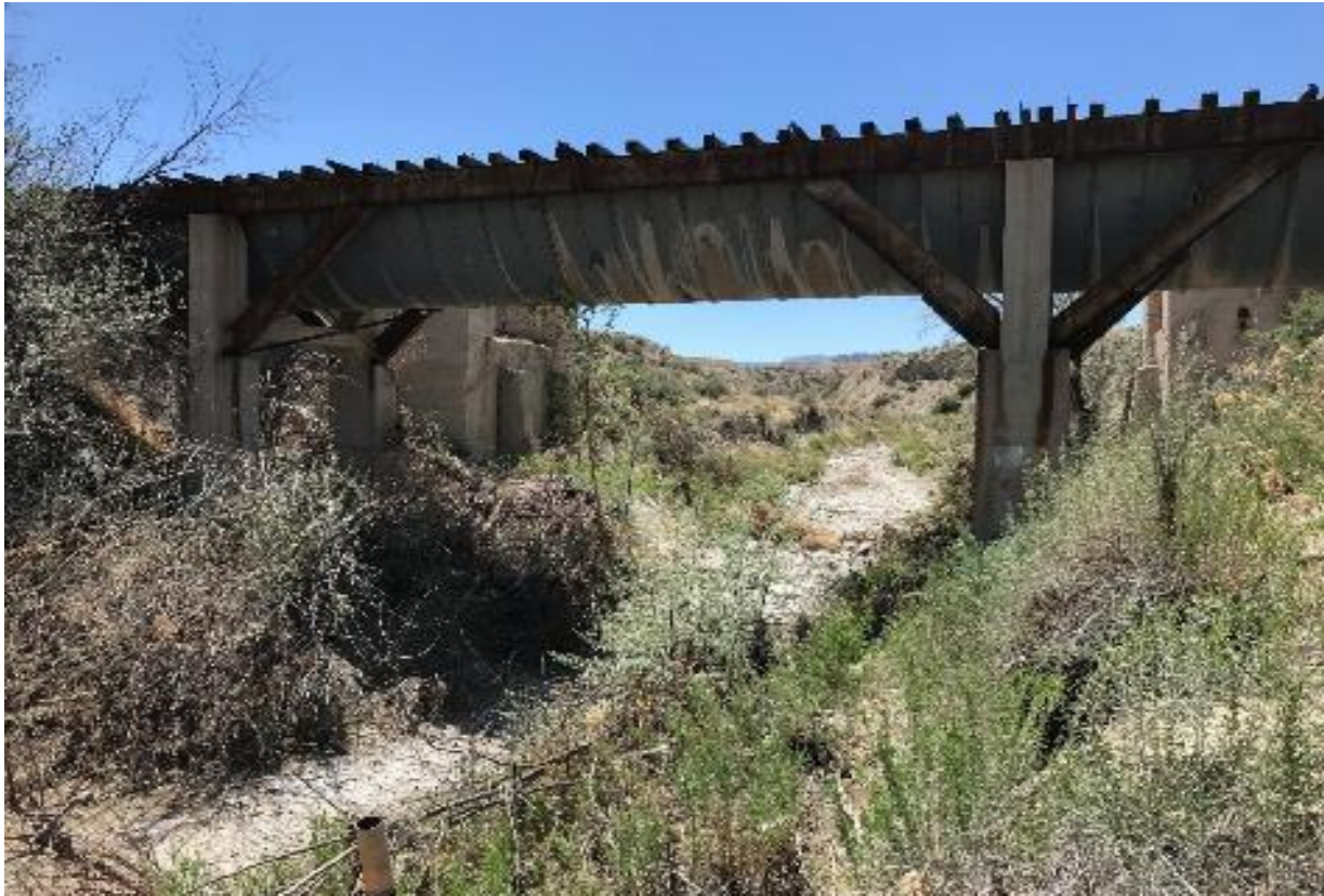
Figure 16. Drunkard's Wash flume side view
