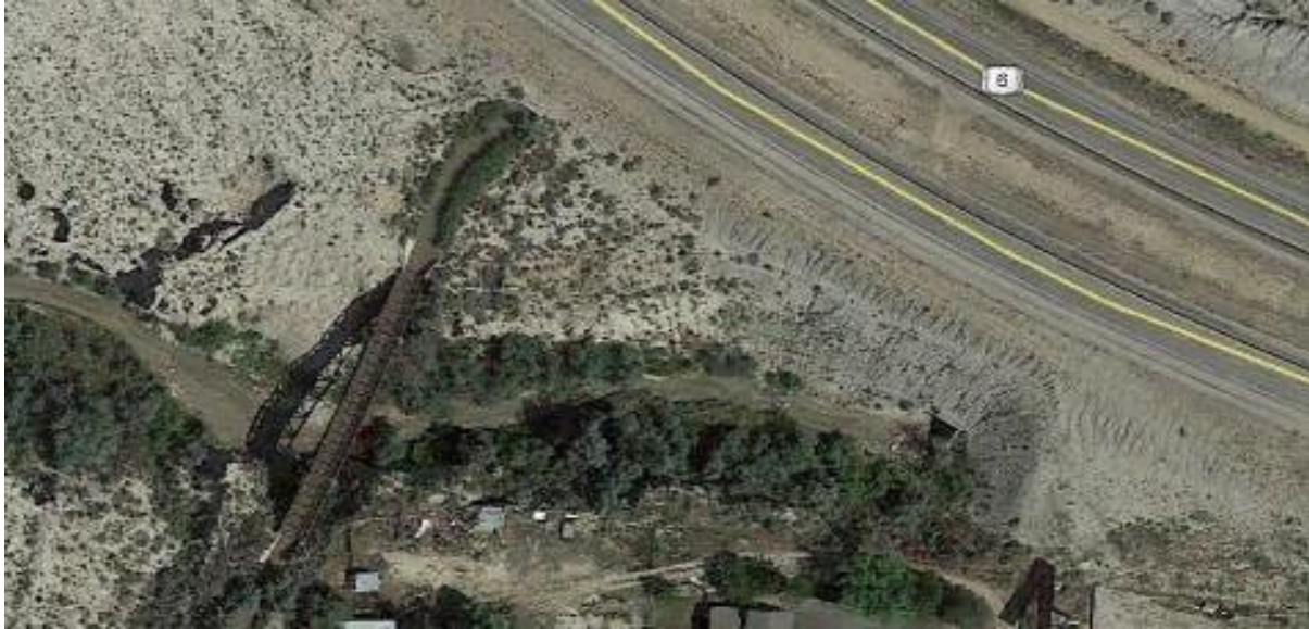
Figure 8. Aerial view of Gordon Creek flume
