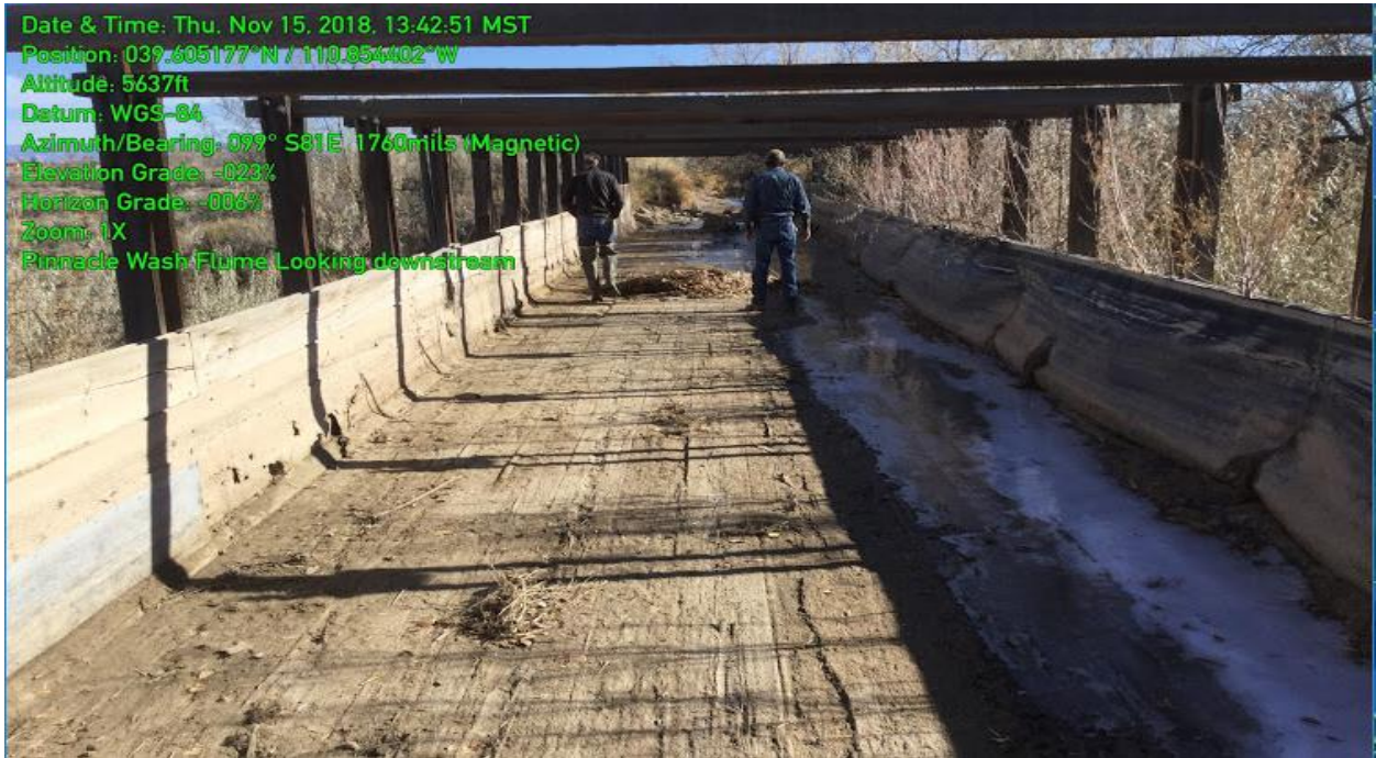
Figure 13. Inside condition of Pinnacle Wash flume
