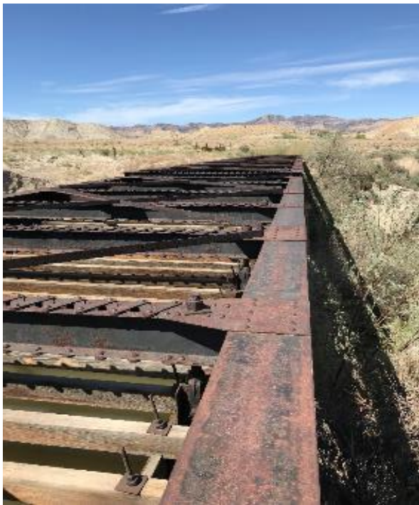
Figure 9. Gordon Creek flume showing girders and cross-braces
