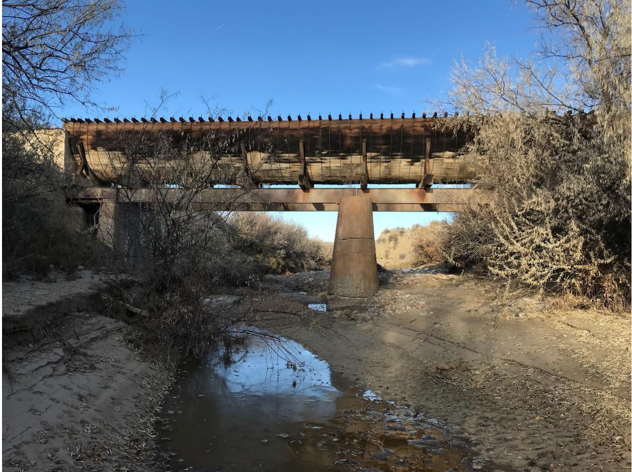
Figure 20. Miller Creek Flume looking west
