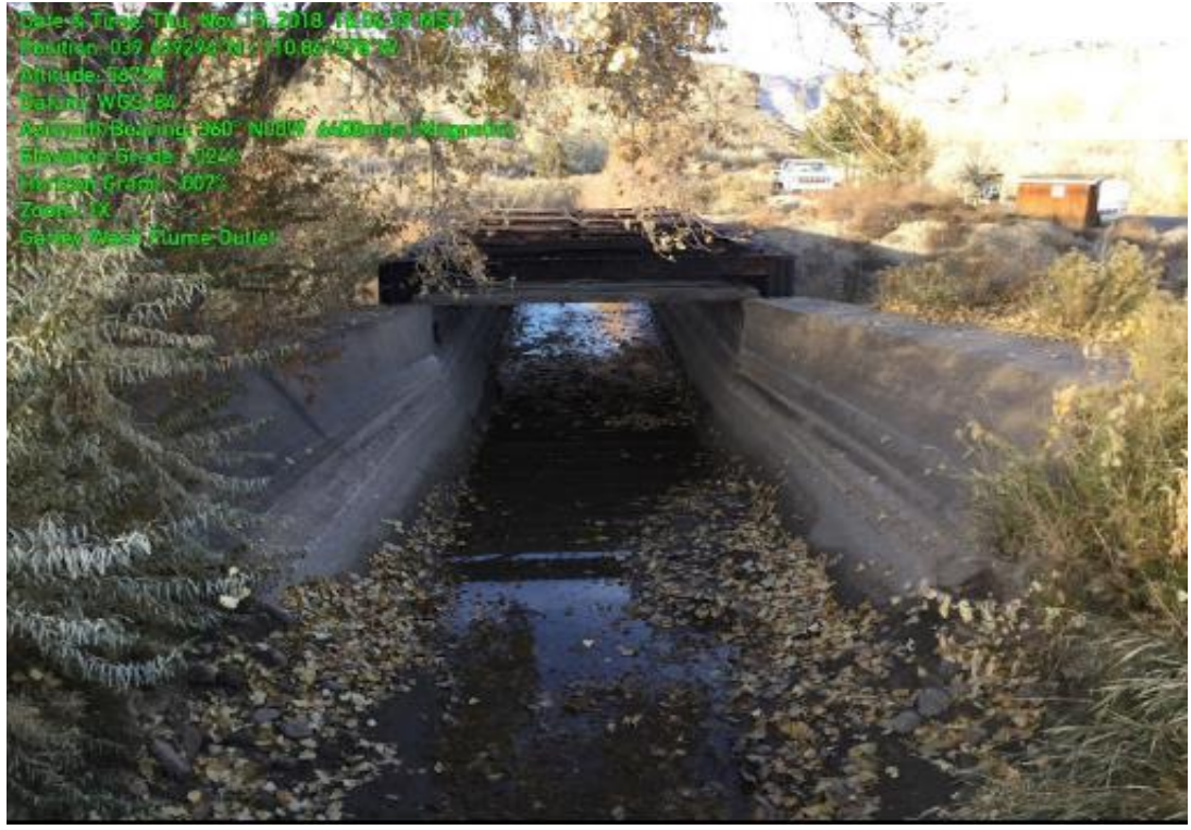
Figure 3. Garley Wash Flume inside view
